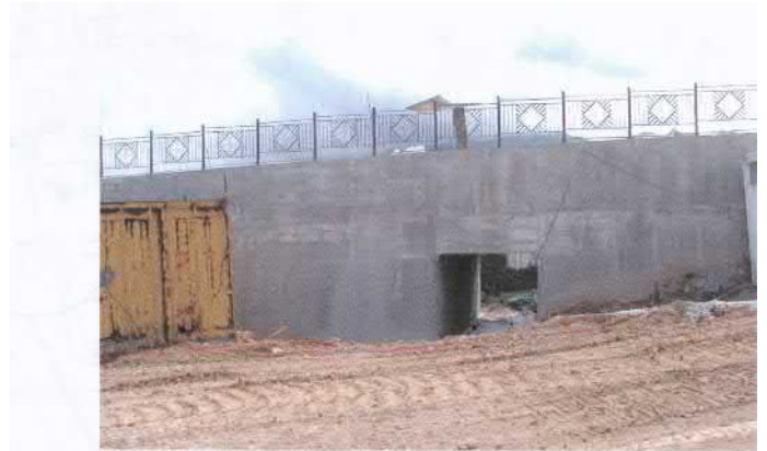
Photo taken on: 22 July 2003 (Front Elevation of the Ramp Structure)
